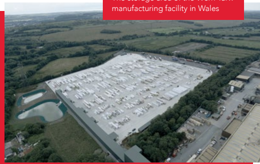
The storage area of the Wern Tarw manufacturing facility in Wales
